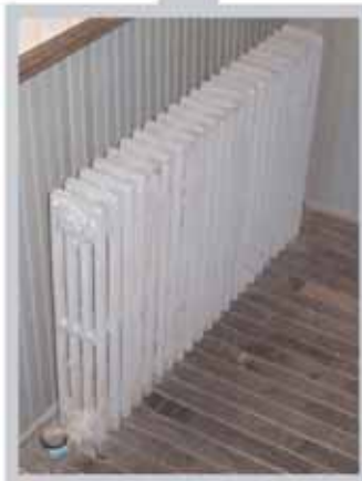
Old style heavy, bulky cast-iron radiators
