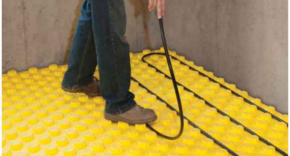
ViegaPEX Barrier tubing in Viega Rapid Grid
