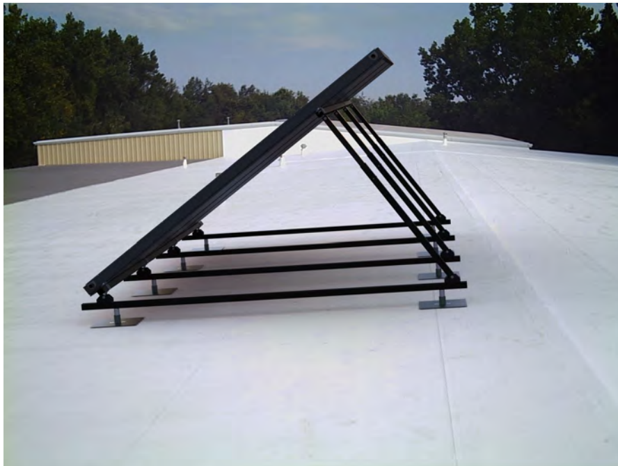
SunEarth RexRack Low Slope Roof Installation
