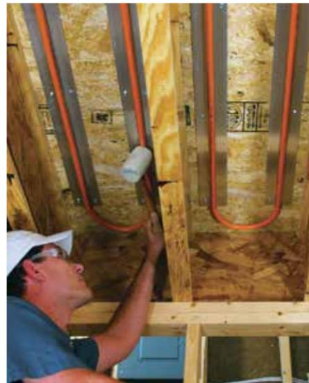
You can install RadiantPEX-AL on the underside of a subfloor, using underfloor plates.
