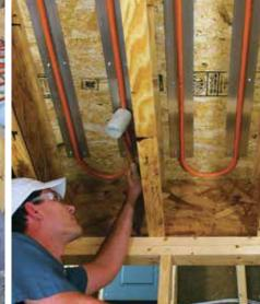
side of a subfloor, using underfloor plates. tie-down easier.
